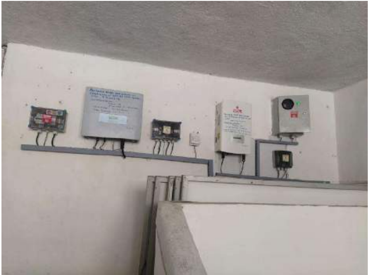
Photo 3- Solar Panel Details Installed
