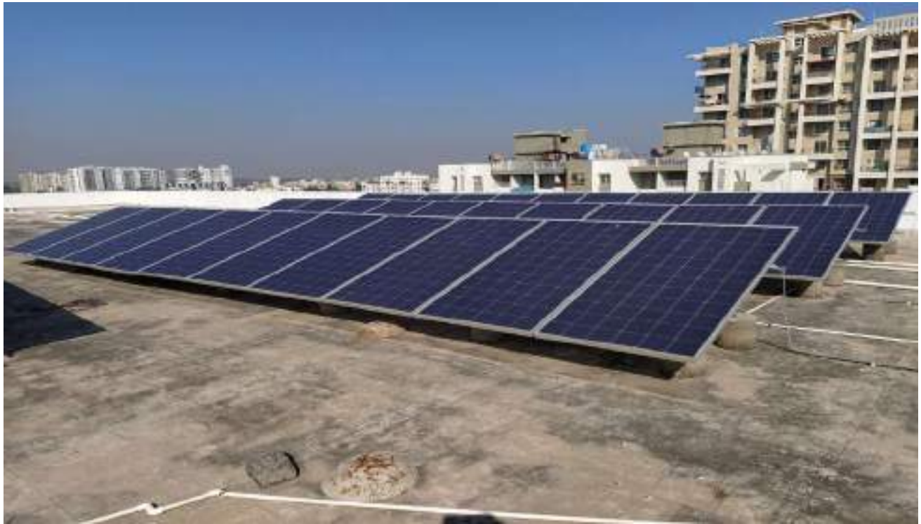
Photo 1: Solar Panel Installed
